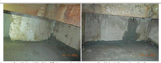
System was found to be visibly dirty. ACs in general can be a source of mold due to the condensation they create and the collection of dirty air. Swab samples can be taken but the solution, if mold spores are present, would be to professionally clean and sanitize the system which should be done with this unit just based on the visible dirt.
