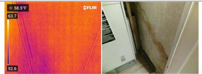
Excessive water staining in furnace closet. No evidence of current moisture. No visible mold present or mildew smells noted. Possibly asbestos acoustic material in closet which should be tested before removing.
