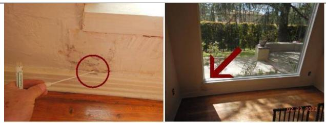
The swab sample showed this mold to be a high level of Ulocladium which takes a good water source to proliferate; outside is found in the soil and decaying plants.
