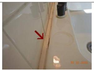
Another source of the mold count could be around the sink. Black staining that appears to be moisture related under/on seal. Recommend removing existing caulk, cleaning, and replace with anti-bacterial silicone.
