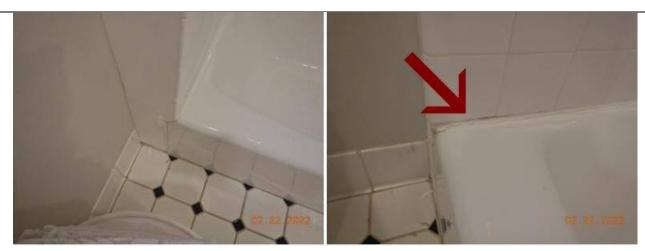
Discoloring noted under caulking which may have been mildew that was cleaned. Recommend removal and replace with an anti-bacterial silicone.
